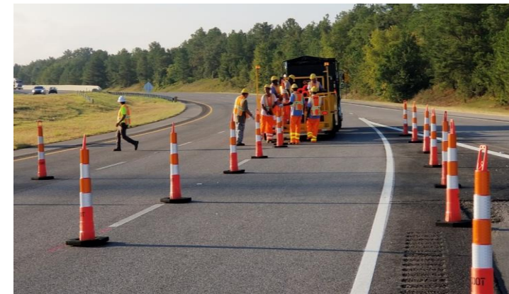
Contraflow traffic operation
